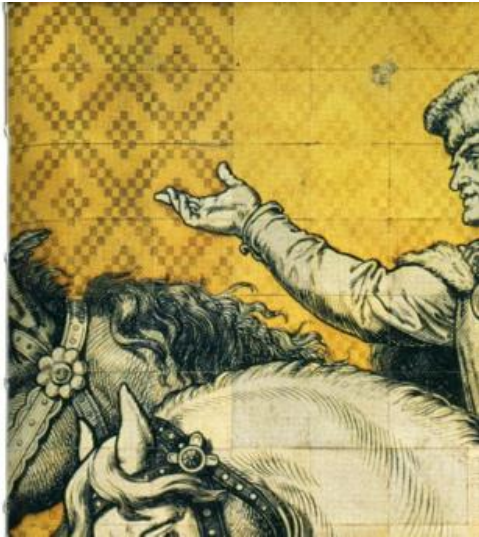
Figure 52. Example of tile discoloration.
