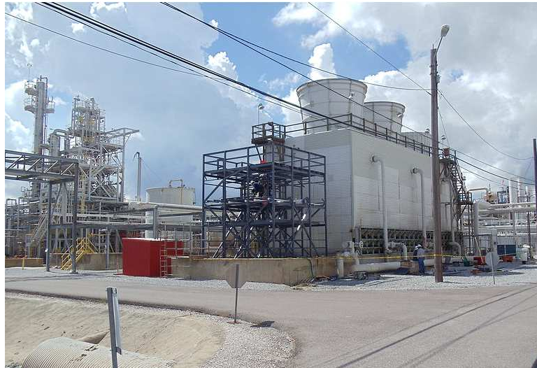
Figure 2-4: FRP Cooling Tower (from Cooling Towers of Texas)
