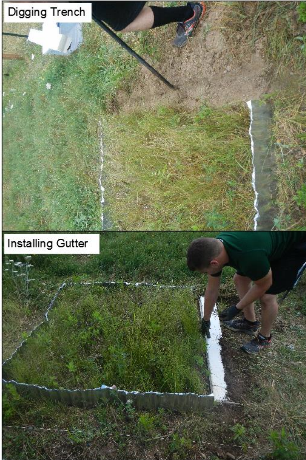
Figure 67: Installation of test sedimentation and runoff collection gutter
