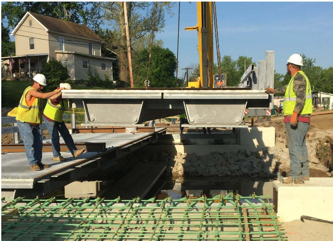
Figure 2.18: Modular SPS Deck/Tub Girder System Being Lowered in Place
