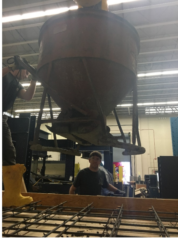
Figure 4.15: Concrete Bucket Lowering into Position
