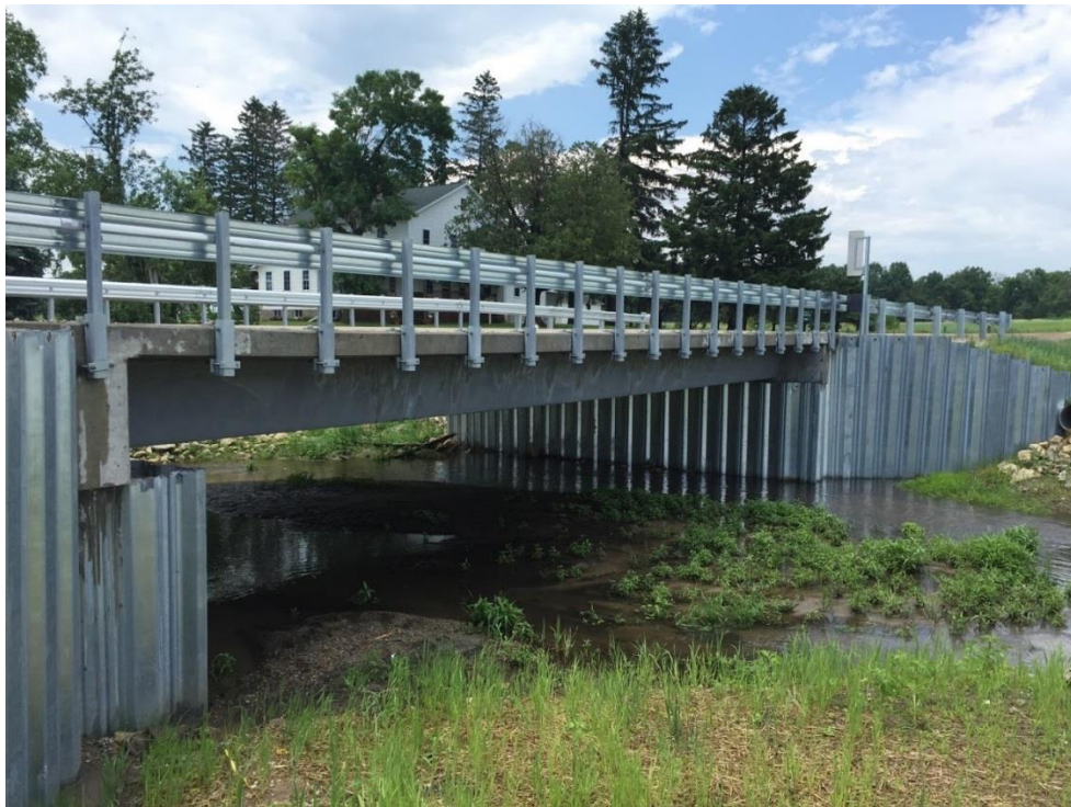
Figure 2.16: New Amish Sawmill Bridge (Gibbs, 2017)
