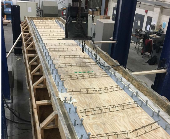
Figure 4.13: Completed Concrete Formwork
