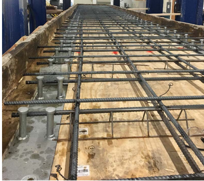
Figure 4.14: Placement of Reinforcing Steel
