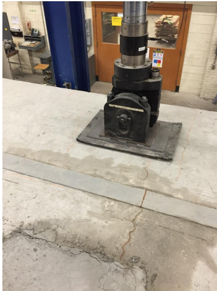
Figure 2.15: Shear Crack Propagated Across UHPC Joint (Kozhokin, 2016)
