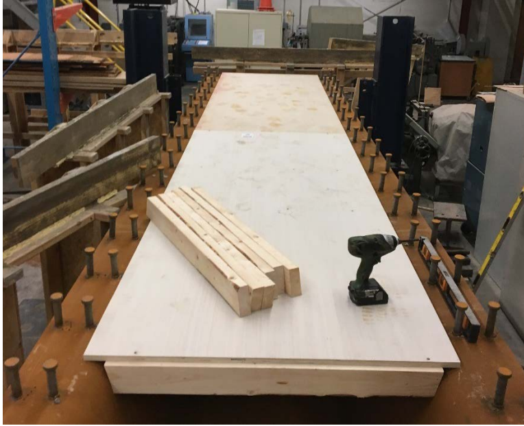
Figure 4.12: Supports Inside the Girder
