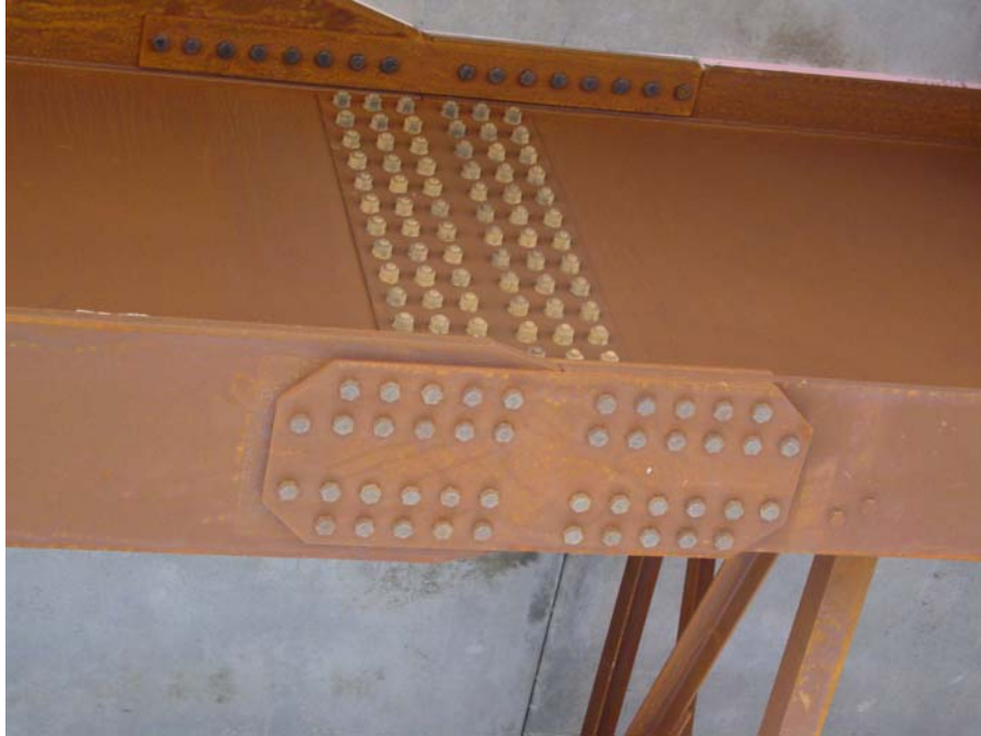
Figure 7.3. Typical field splice
