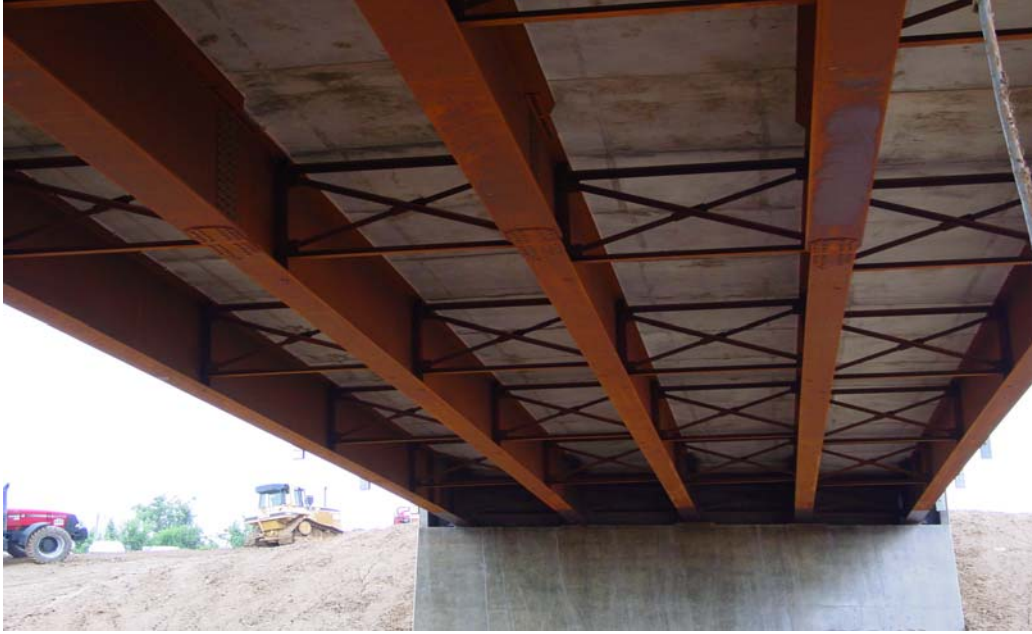
Figure 7.2. Underside of Missouri Bridge A6101
