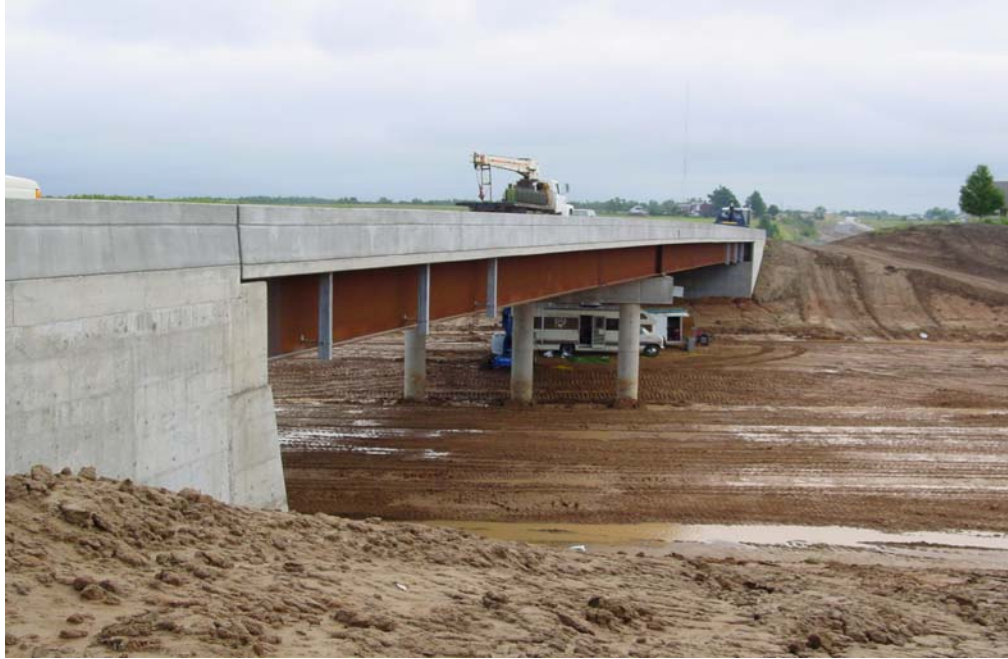
Figure 7.1. Elevation of field-tested/Missouri Bridge A6101
