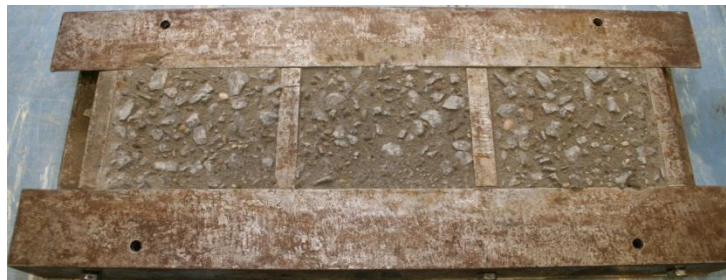
Figure 6.5 Mechanically prepared substrate surface
