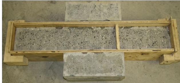
Figure 6.39 Formwork for pouring of repair material
