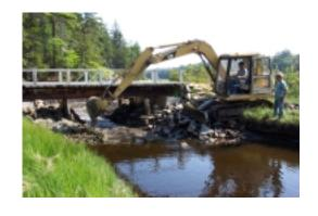
and Bates College have collaborated to develop and fund restoration and follow-up monitoring. Preliminary engineering work confirmed the need to remove 100 cubic yards of rock from under a bridge to eliminate the tidal constriction and the need to prevent excessive drainage.
