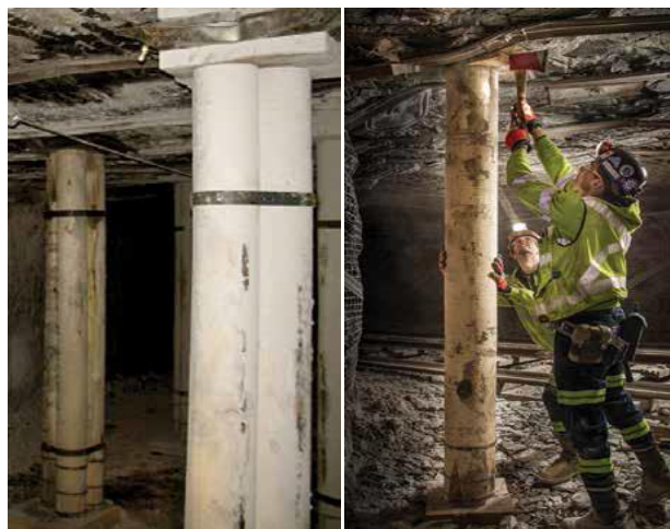
Figure 2-6 Prosetter and Cluster support in underground mine (Strata web, 2014)
