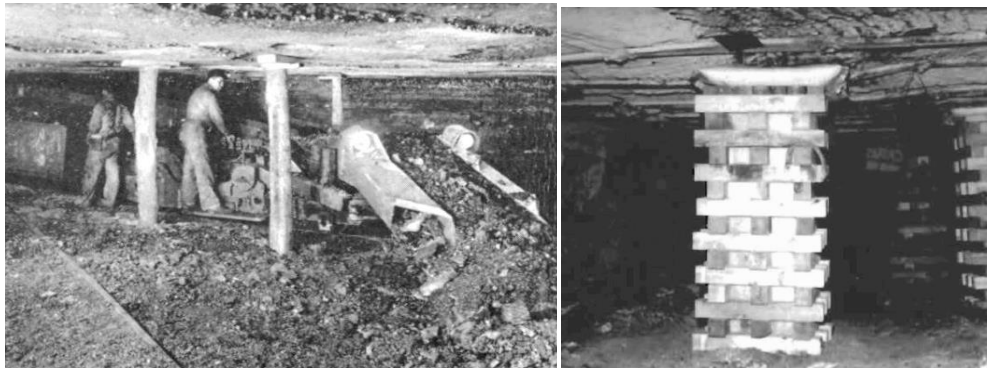
Figure 2-5 Wood cribs in bleeder area (C. Mark, 2002)
