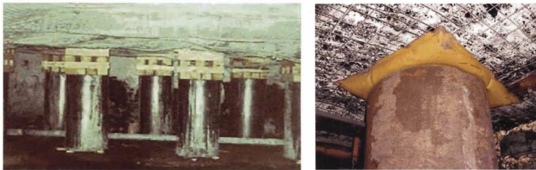
Figure 2-7 Can support and the Prestressing Units (T.M. Barczak, 2006)
