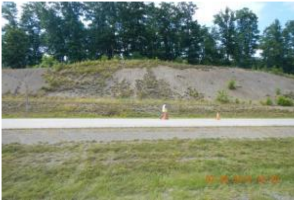
Figure 19: Corridor H Site 2A
