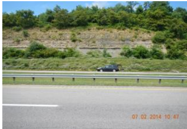
Figure 14: Mon-Fayette Expressway Site 1
