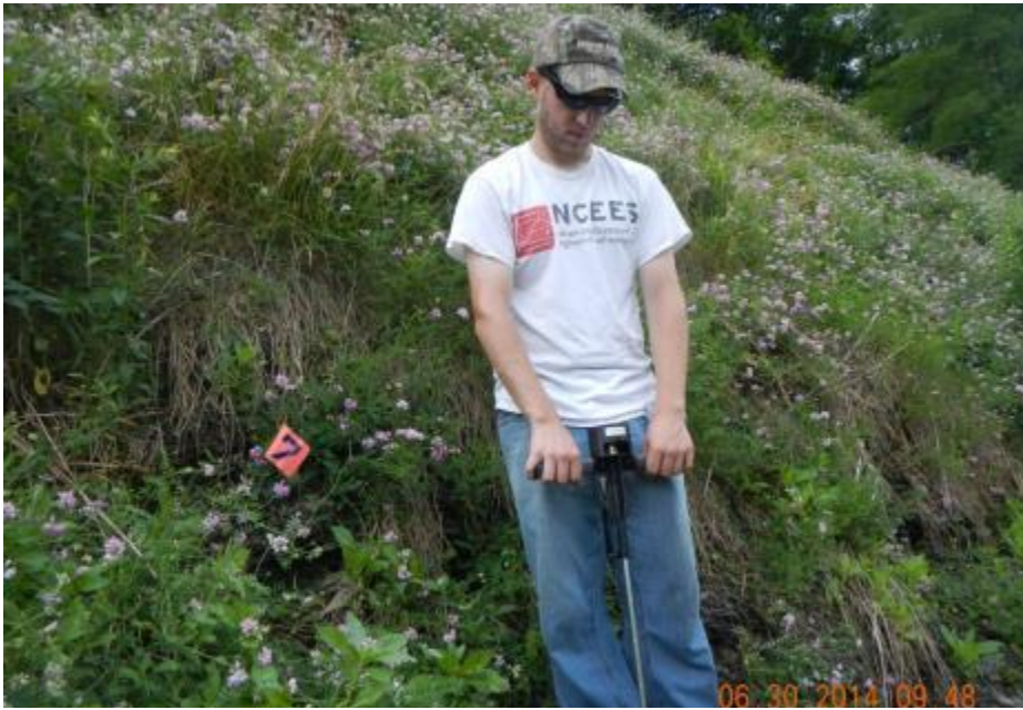
Figure 60: Compaction testing at Philippi Bypass
