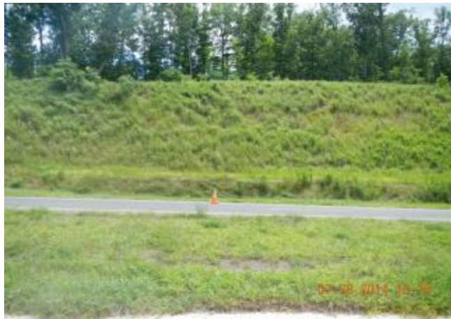
Figure 23: Corridor H Site 5
