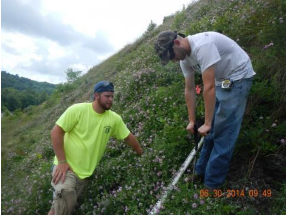
Figure 61: Compaction testing with penetrometer at Philippi Bypass
