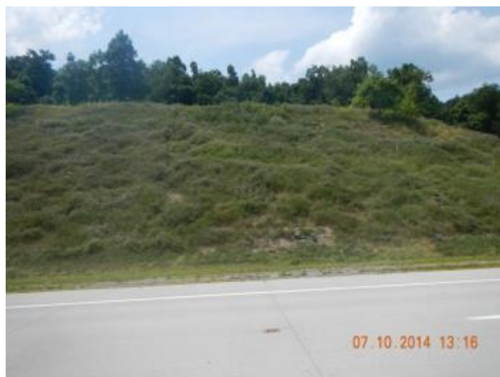
Figure 20: Corridor H Site 3
