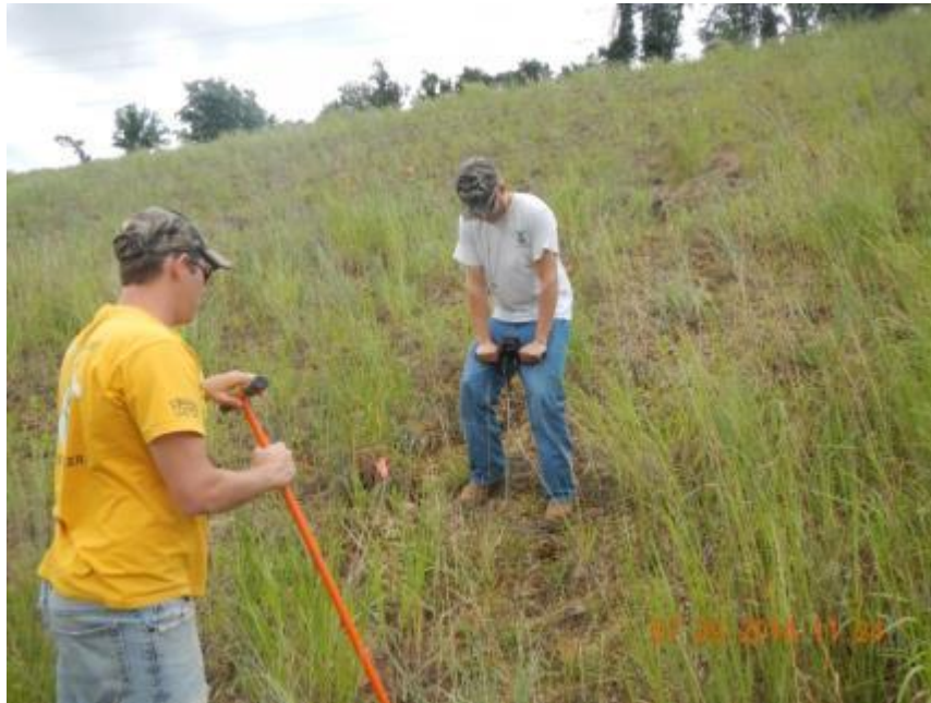
Figure 82: Compaction testing with penetrometer at Route 9 Site 1
