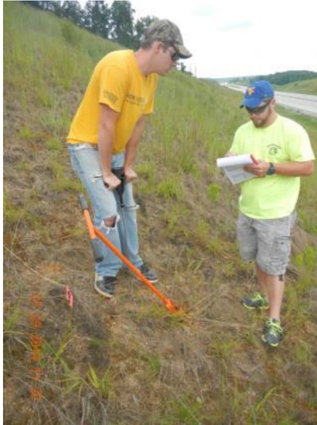
Figure 83: Compaction testing with penetrometer at Route 9 Site 1
