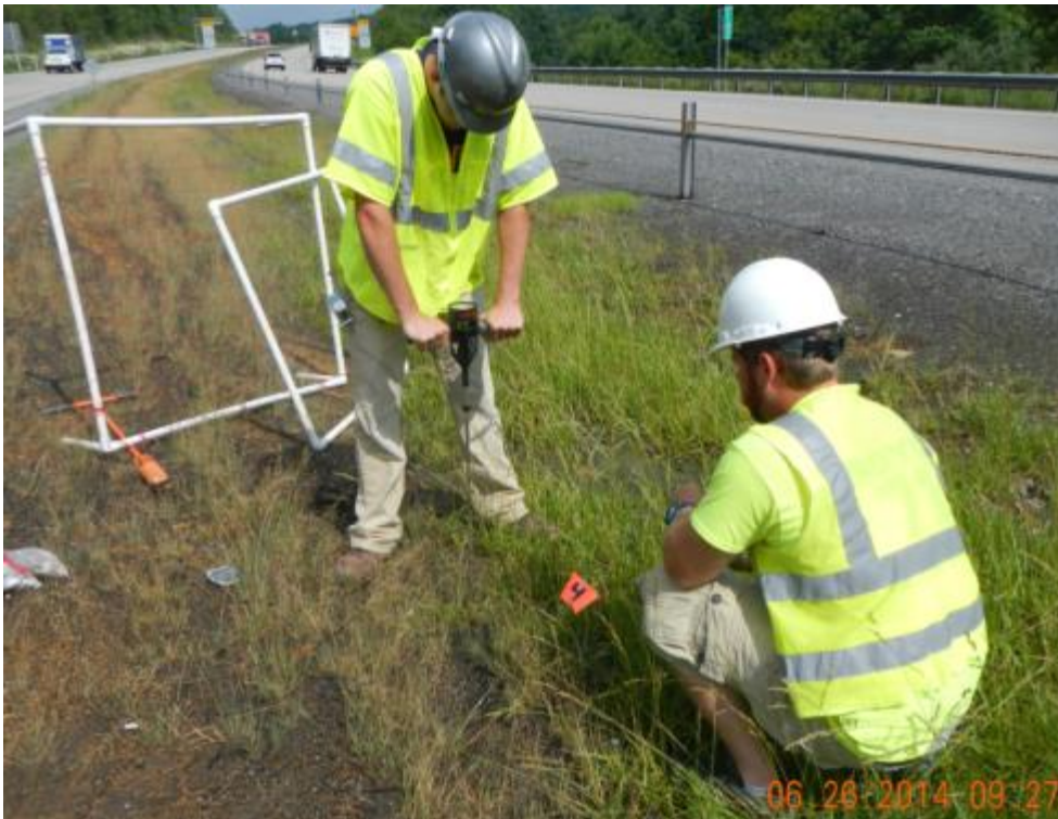
Figure 56: Compaction testing with penetrometer at I-68 median
