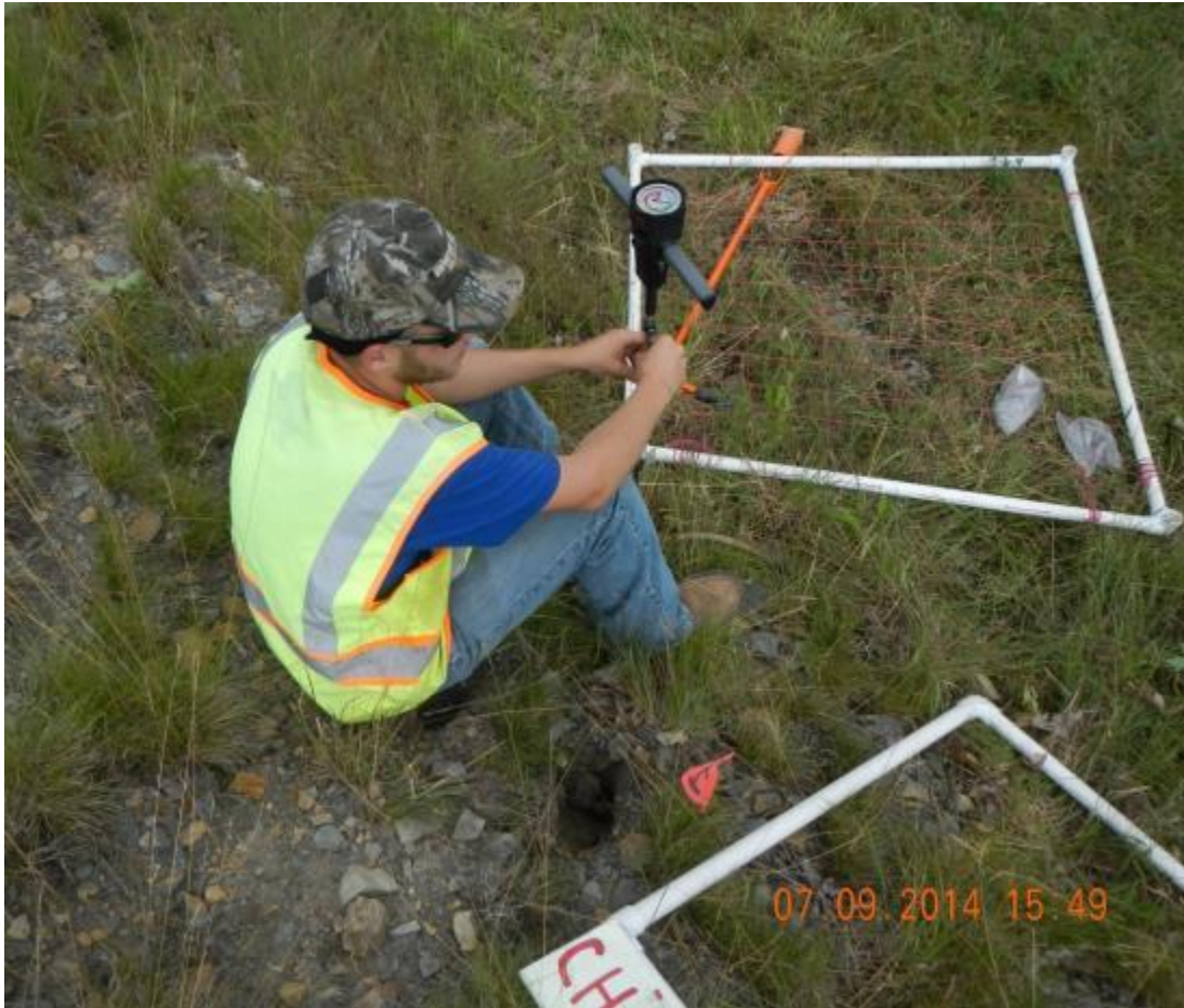
Figure 69: Preparing for compaction test at Corridor H Site 2
