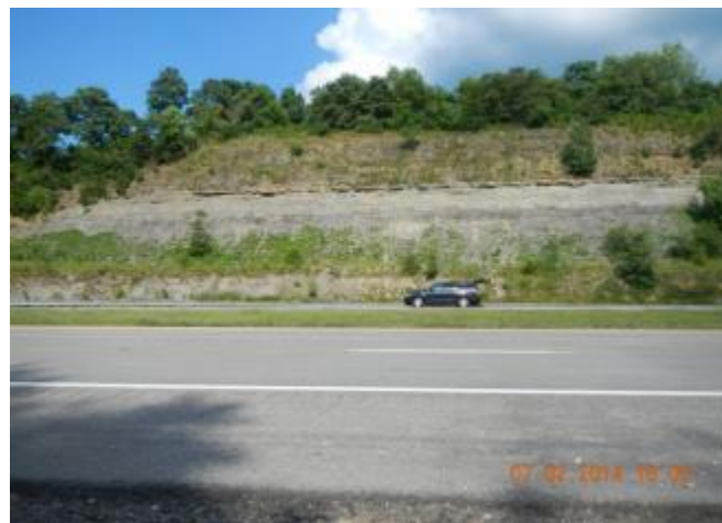
Figure 15: Mon-Fayette Expressway Site 2
