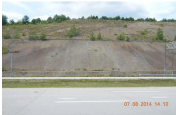
Figure 16: Corridor H Site 1
