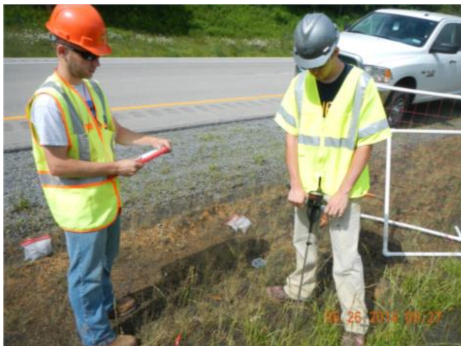
Figure 54: Soil compaction testing with penetrometer at I-68 median
