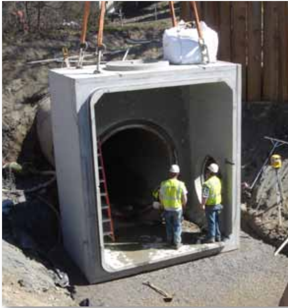
Baxter Boulevard CSD storage conduit during installation.
