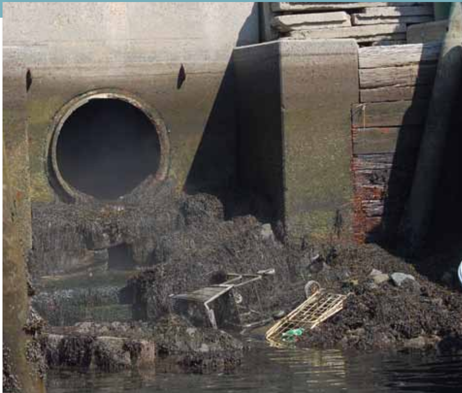
CSO discharge point on the Portland waterfront, adjacent to the Casco Bay Ferry Terminal.
