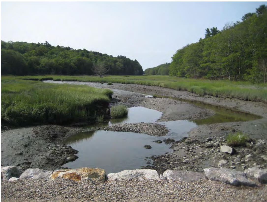
View of channel and scour pool upstream of culvert inlet.
