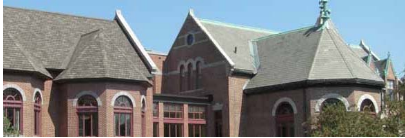
AUBURN LIBRARY, original structure on right, circa 1904. Addition on left, circa 2006.
