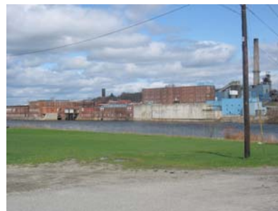
MILL COMPLEX IN WATERVILLE
