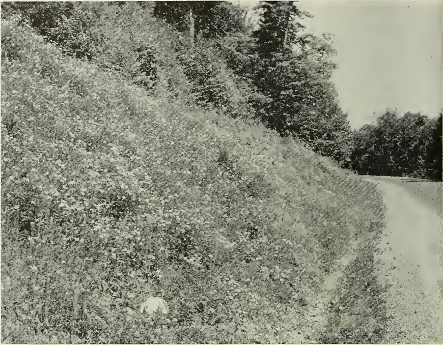
FIGURE 7. One-year-old seeding of crownvetch on roadbank on W. Va. Route 39, about eight miles west of Mill Point. The bank was bare when seeded. The site, with an elevation of 3,928 feet, was selected to evaluate winter hardiness of crownvetch.
