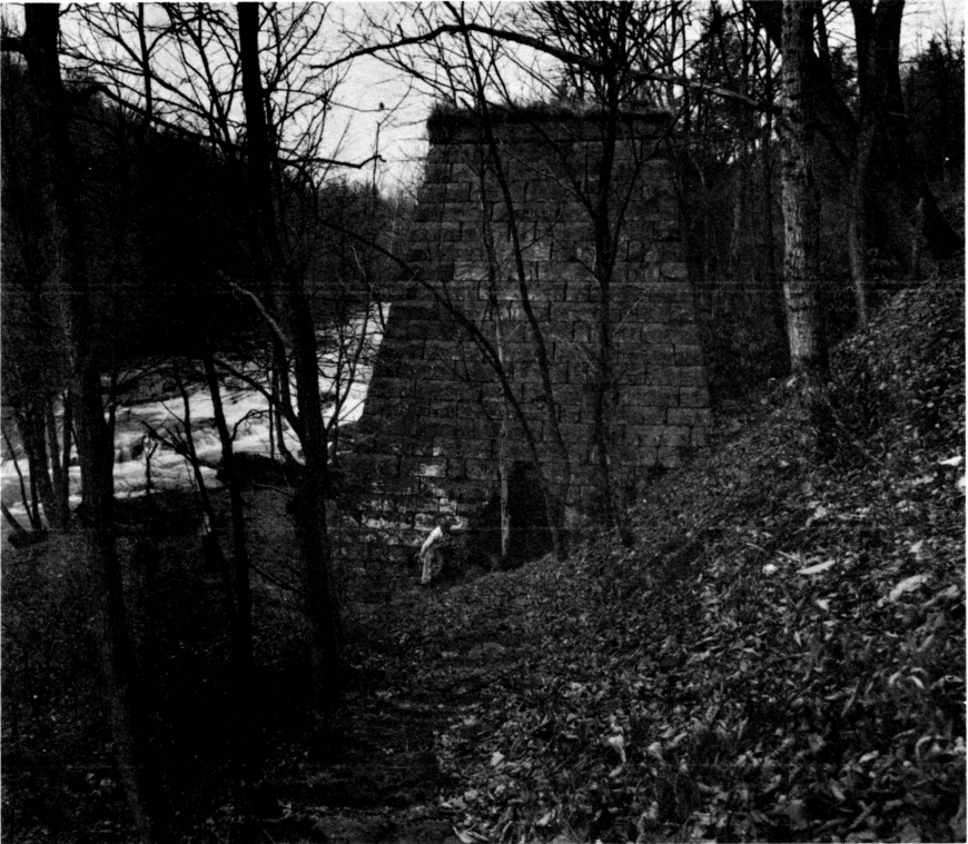
Figure 3. Iron furnace restored.
