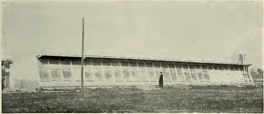
FIGURE 11. The New Jersey experimental solar poultry house. This house will maintain excellent litter with the equivalent of one Leghorn layer per two square feet of floor area. The six easterly panels on this house are covered with plywood. Experimental work was done with an uninsulated house 30 feet in width.
