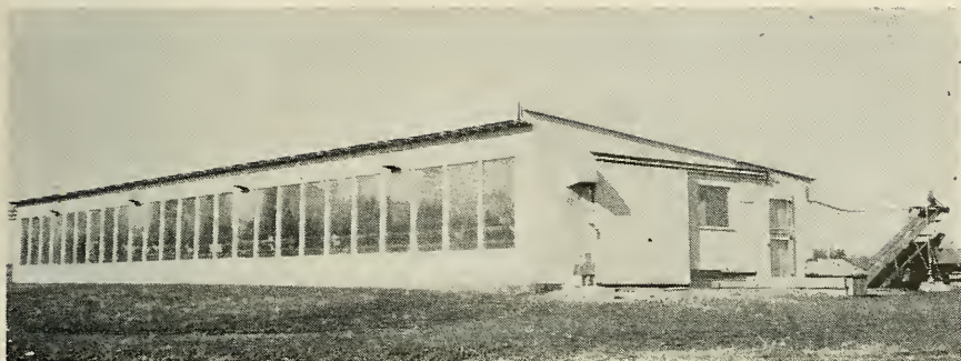
FIGURE 8. Experimental solar poultry house at the Pennsylvania Station. This 30-by 100-foot house has two inches of Fiberglas insulation in the walls, and four inches in the ceiling. The vapor barrier is aluminum foil. The concrete floor is also equipped with a vapor barrier. Insulating-glass windows are exposed due south. The ventilation system consists of thermostatically-controlled pressurized inlet fans.
