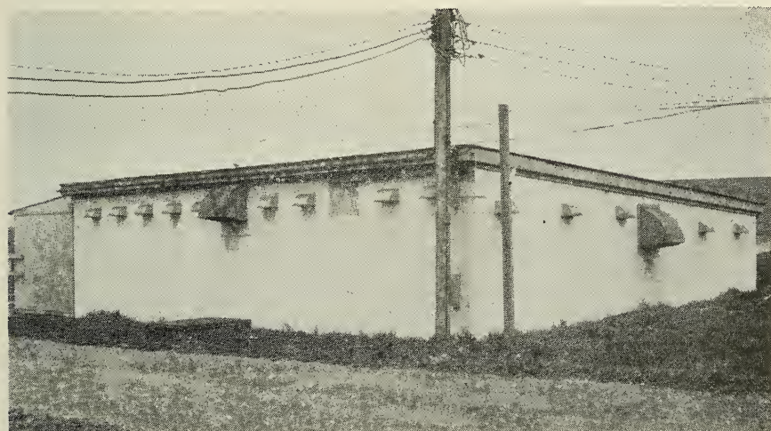
FIGURE 10. The experimental windowless house at the West Virginia University Agricultural Experiment Station, with a floor area of 900 square feet, is constructed of cinder blocks. Cores are filled with expanded vermiculite.
