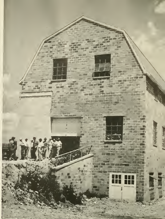
NEW BUILDINGS and installations are featured on Field Day programs. Visiting poultrymen inspect feed-mixing facilities at Reymann Farms.
