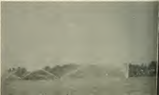
IRRIGATION system, installed at the Reymann Memorial Experimental Farms, provides water for crops during dry seasons.
