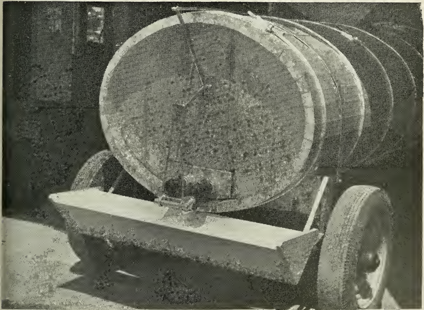
FIGURE 6. Rear view of 500-gallon tank with 6-foot trough. Valves are controlled by levers at front of the wagon. Holes in trough help provide even distribution.
