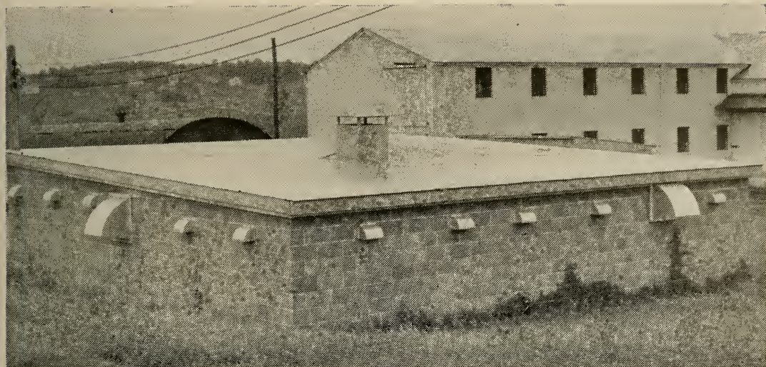
FIGURE 1. Windowless house showing original ventilation system of 24-inch exhaust fan in center of roof and small, hooded intake openings. This system was discarded in favor of a pressurized system. The large hoods in the walls cover the intake fans and exhaust openings.
