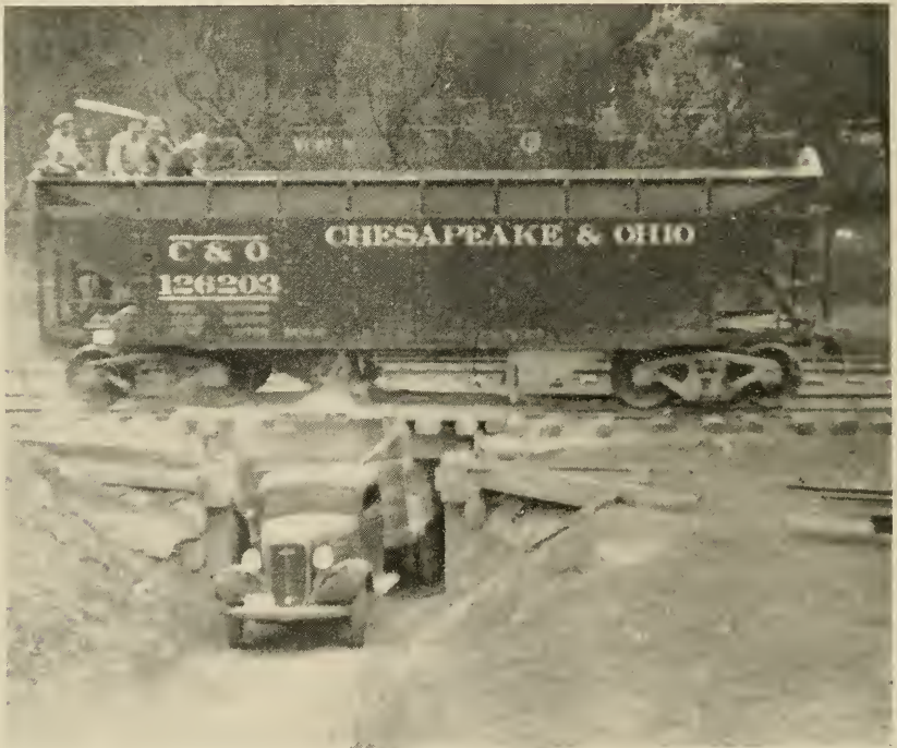
An inexpensive method of unloading high-sided, hopper-bottom cars. Where no underpass can be arranged, a belt conveyor (with one end in a shallow pit dug out underneath the railroad, the other end elevated over the truck bed) proves a big labor saver where a sufficient quantity is to be unloaded.
