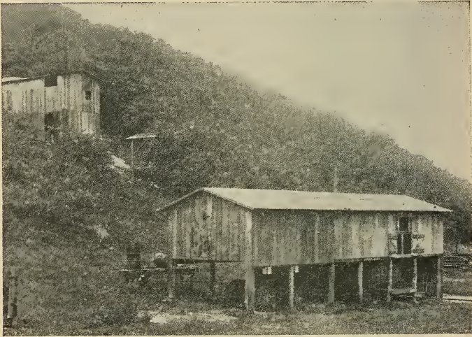
Central plant of a stationary spray system on a large orchard
