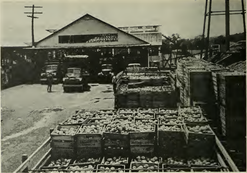
APPLES arriving at receiving station of processing plant.
