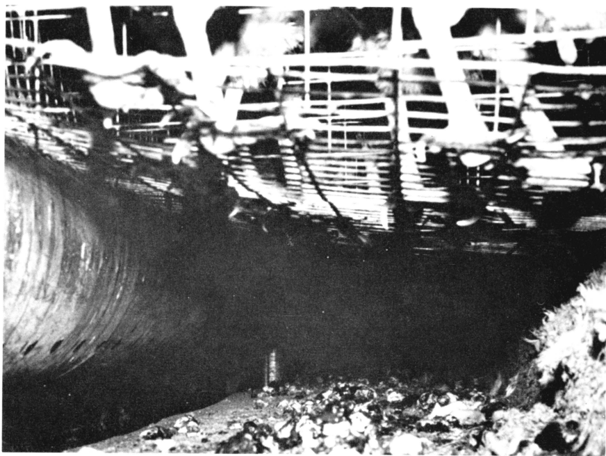
Figure 3. Air Duct with Air Jets in Operation
