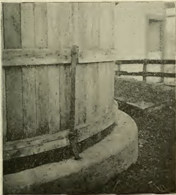
Fig. 7.—Anchor Irons Set in Foundation.
