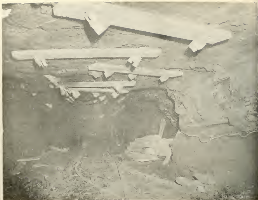
Figure 2. Suspension timbering using wood mine pins and cross-headers. Courtesy of U.S. Bureau of Mines
