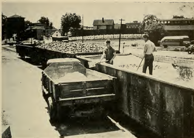
Fig. 2—Unloading ground limestone at Buckhannon for use in connection with the Agricultural Conservation Program
