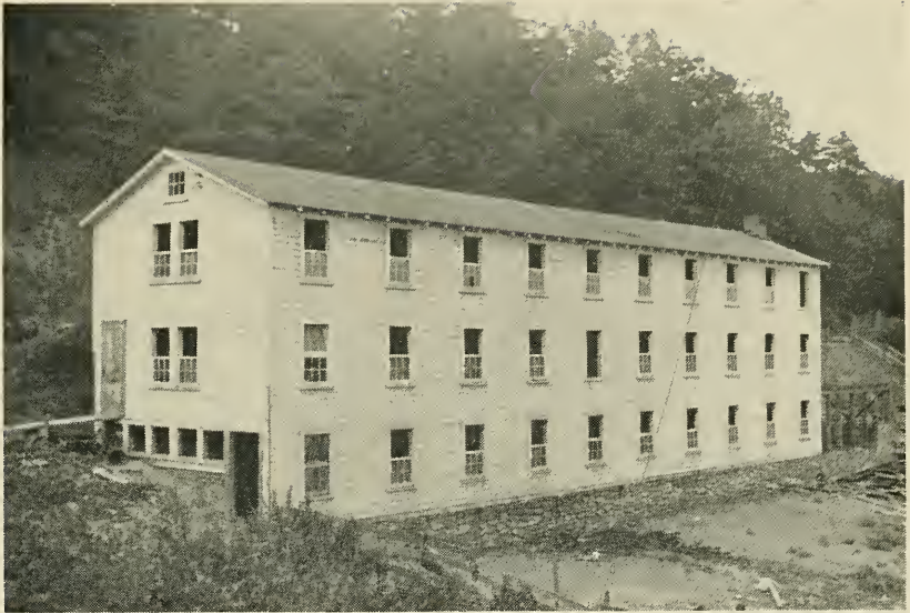
Fig. 6—Three-story Broiler House Constructed from Locally Sawn Timber. Second and Third Floors Are Wood and the First Concrete. This House of 5000 Capacity Was Heated by a Furnace and Was Constructed at Moderate Cost
