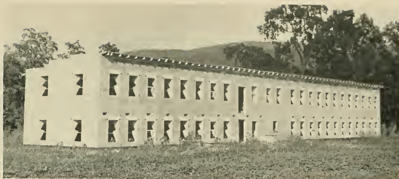
Fig. 7—Two-story Broiler House Constructed from Concrete Blocks. This House of 5000 Capacity Had a Dirt Floor on the Ground Level and a Concrete Second Floor. It Was Heated by a Furnace and Was in the High-construction-cost Group
