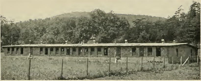
Fig. 8—Broiler House Constructed from Cinder Blocks. This House of 5000 Capacity Had a Dirt Floor and Was Heated by Wood Brooder Stoves. It Was Built at Moderate Cost
