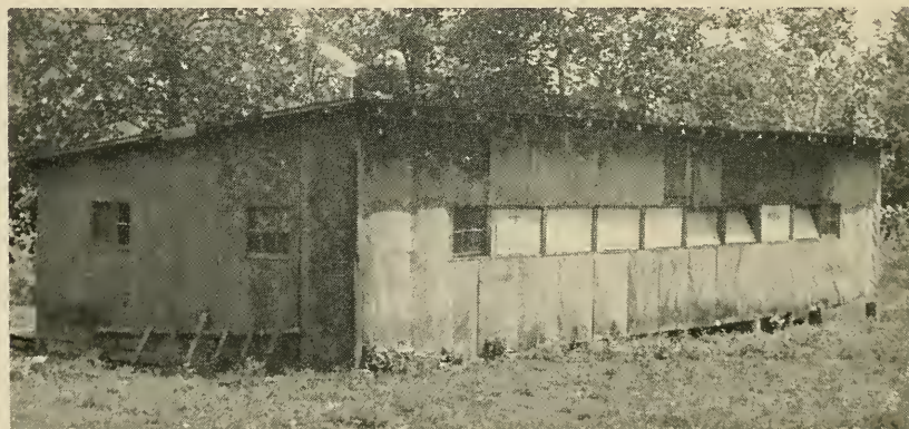
Fig. 5—Broiler House Constructed from Locally Available Rough Lumber and Roofing Material. It Had a Wood Floor and Was Heated by Wood Brooder Stoves. The House Had a Capacity of 900 to 1000 Broilers and Was Constructed at Relatively Low Cost. Building Cost Could Have Been Reduced Still Further by Omitting the Wood Floor
