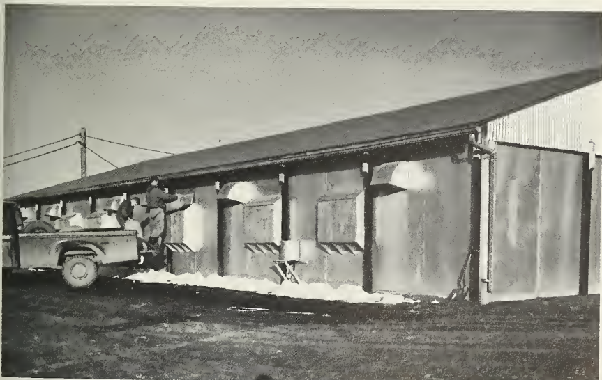
FIGURE 7. This is the west side of the broiler house, showing air intake fans, feed hoppers, and fuel supply for the brooder units.
