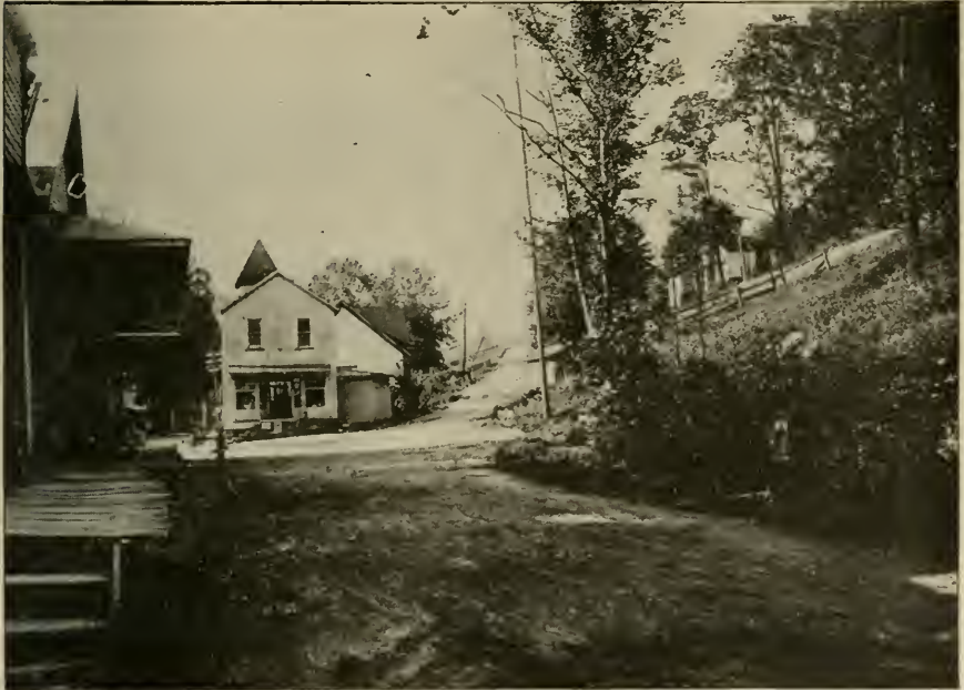
A view of the principal street in French Creek village. Arrangements have been completed for the construction of concrete sidewalks along this street. Such evidence of community spirit adds to the score under "Business."
