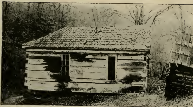
One of the old pioneer log cabin homes of French Creek.
