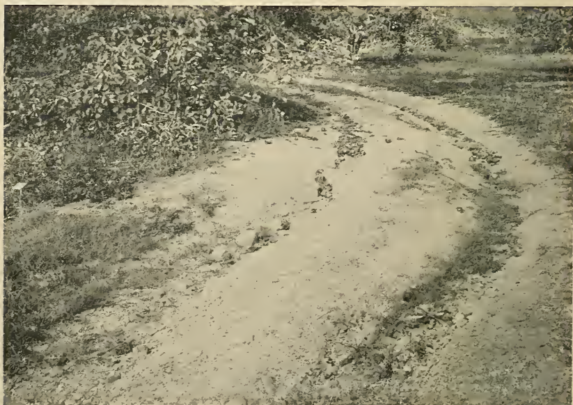
Fig. 3—An orchard road on the Berks. The wheel tracks erode typically with nearly vertical sides. They may become so deep that the axles and under-carriages of orchard machinery drag, thus forcing either extensive repairs or abandonment of the road
