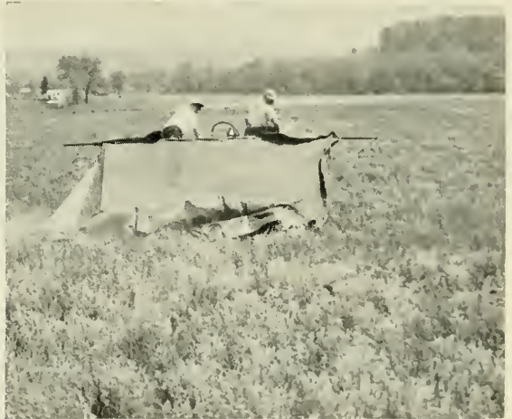
Figure 1. Air siphon type ULV sprayer used in the 1965 experiments.
