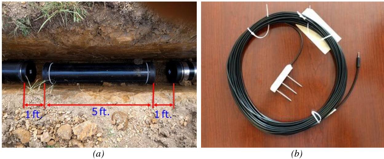
Figure 6-14: (a) Arrangement of pipes in the trench, (b) soil moisture and resistivity sensor
