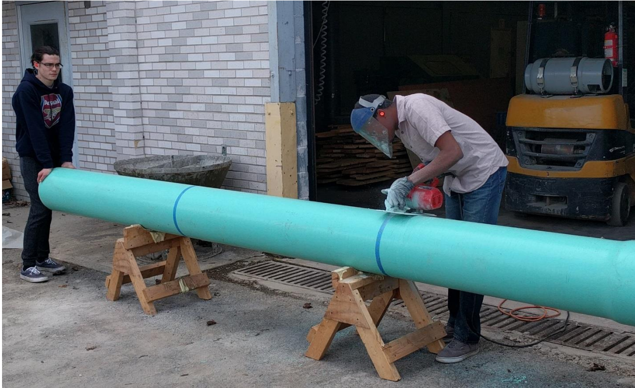
Figure 6-1: The 14' long 12" diameter PVC pipe being cut
