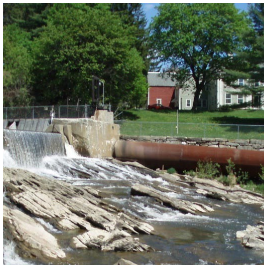
Bridge Street Dam Head Gate Structure and Sparhawk Mill Penstock
