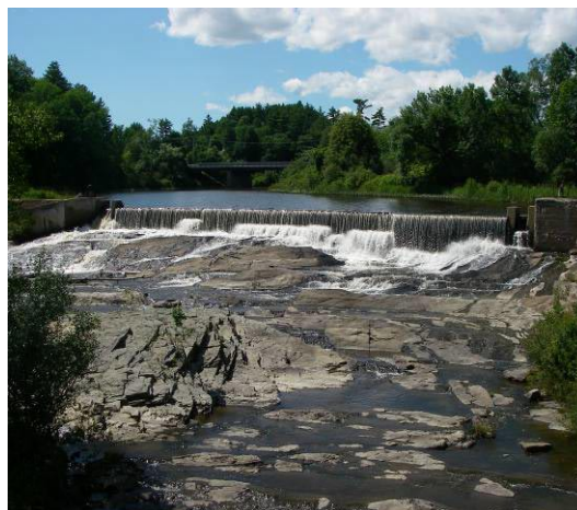
Bridge Street Dam as viewed from north side of the Bridge Street bridge
