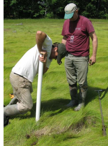
Photo 3. Installing a deep water monitoring well.
