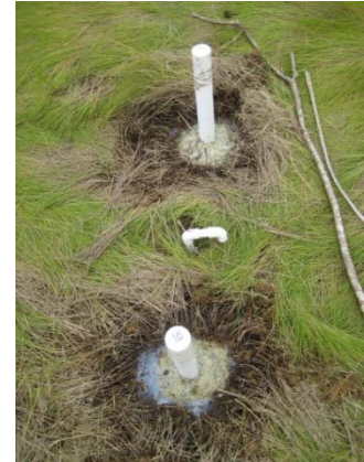
Photo 2. Typical cluster of Station wells.
