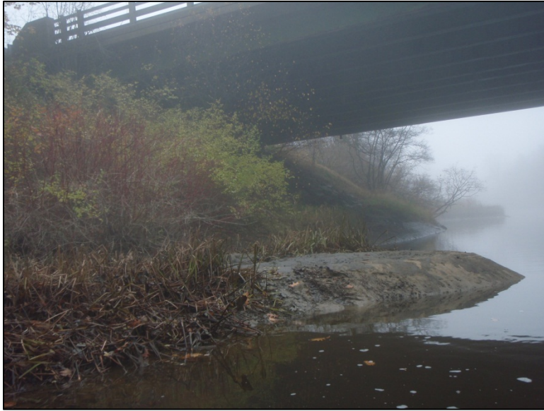
Photo 2: Accumulated Sediment at Stormwater Outfall (left side of river immediately upstream from U.S. Route 1 Bridge)
