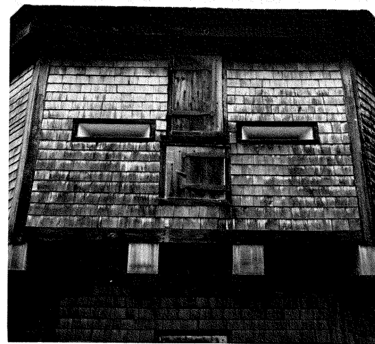
36. Fort Edgecomb blockhouse, detail
