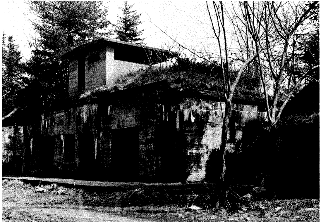
57. Fort Baldwin, Battery Hardman from the rear
