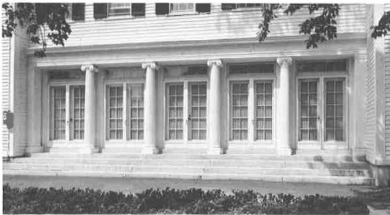
The colonnade on the south facade designed by John Calvin Stevens in 1919.
