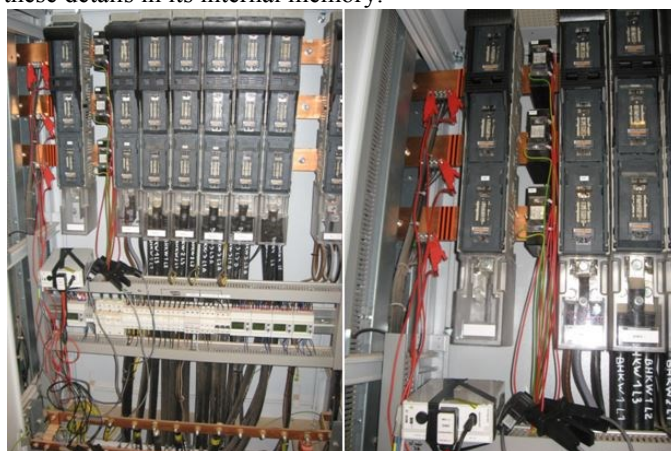
Fig. 1. Demonstration of a connection measurement equipment in the BS 1
