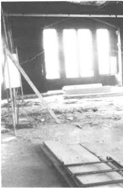
Corthell Concert Hall renovations, 1985.
