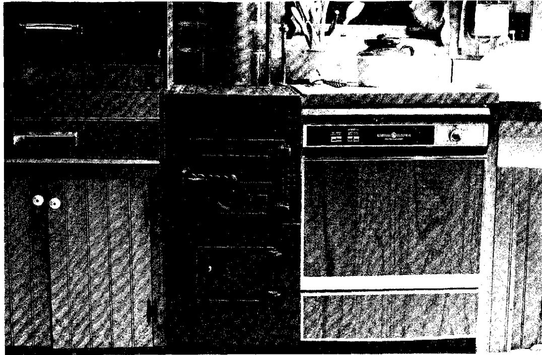
■ Mr. Lund's stove installed in a kitchen counter. The sides and back are cooled by convective air currents.
