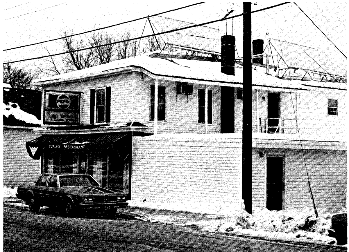
Roof-mounted Solar Water Heating Panels.
