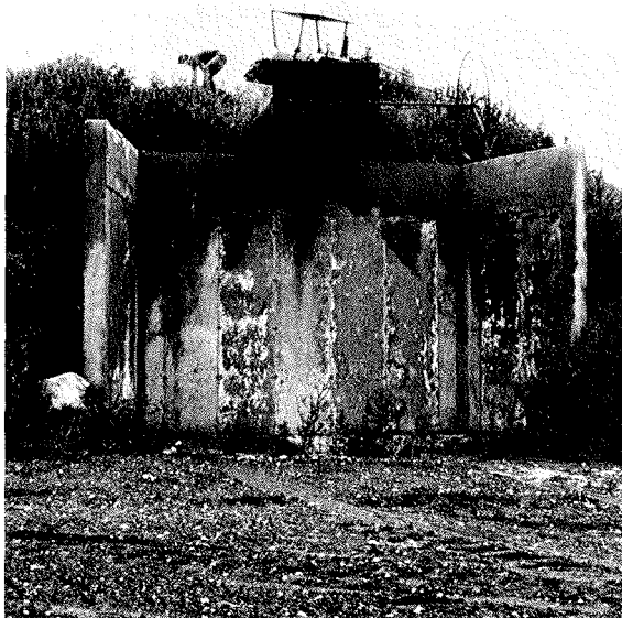
14. Gravity flow manure storage at Carrier's saves time and energy
