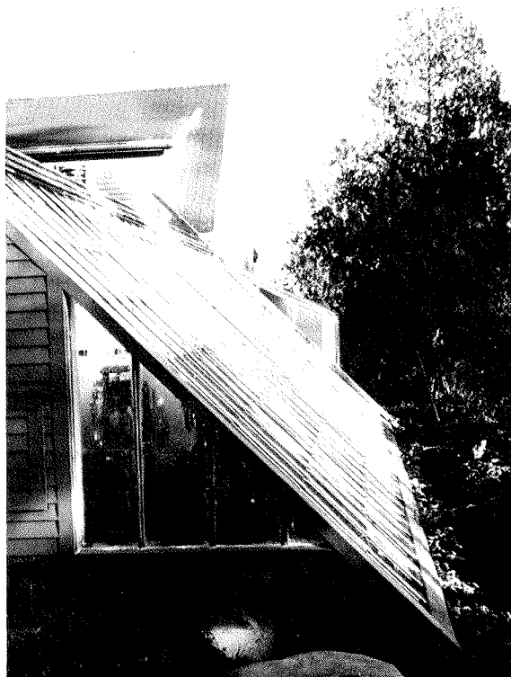
11. Whitney's solar greenhouse utilizes double glazing and a 2-foot rock bottom for heat storage
