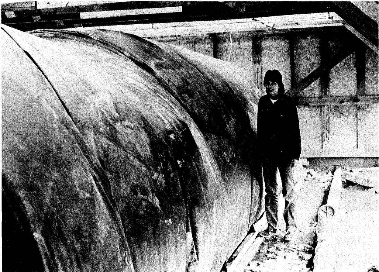
22. Tait's digester with gas bag fully inflated
