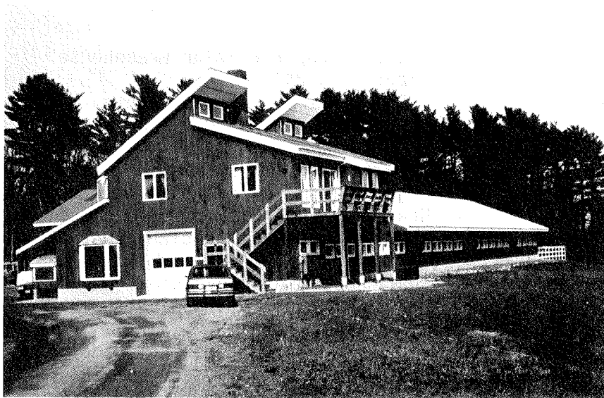
10. New solar barn at Smiling Hill Farm
