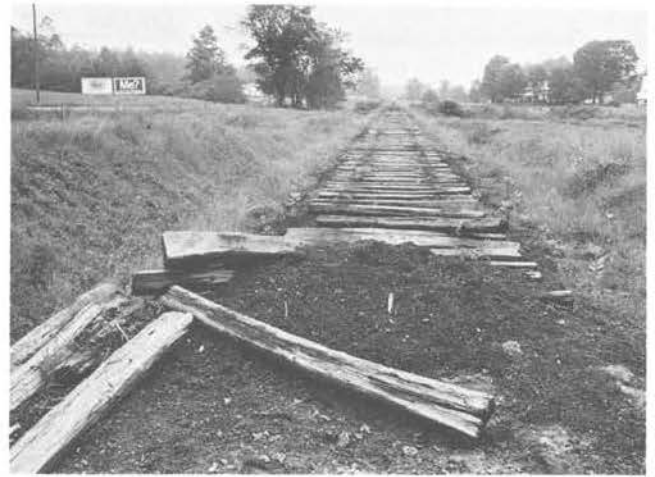
ABANDONED GRADE WITH TRACK DOWN
