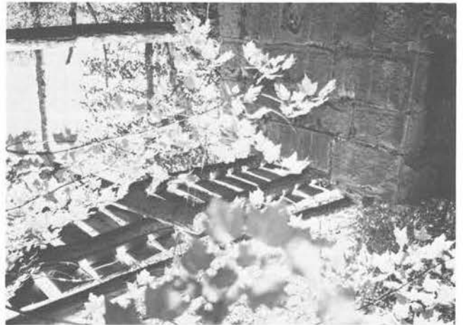
SIMPLE FOOTBRIDGE CONSTRUCTION
