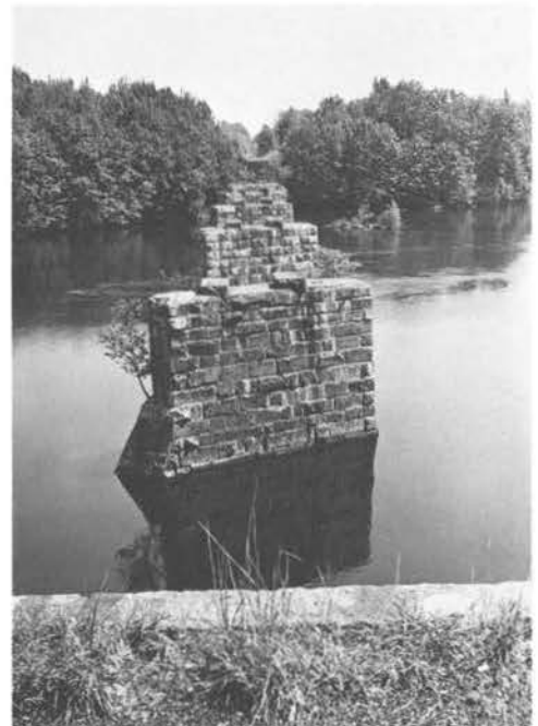
TRESTLE PIERS OVER SACO RIVER, BAR MILLS
