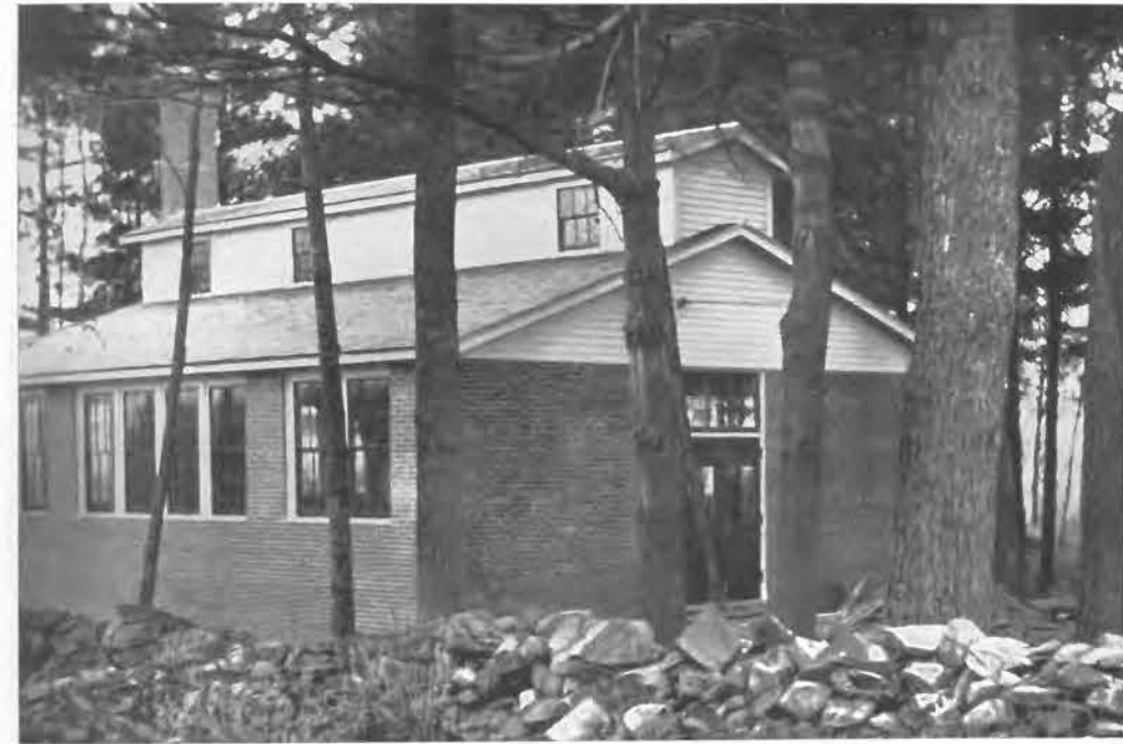
FORGE AND MACHINE SHOP
