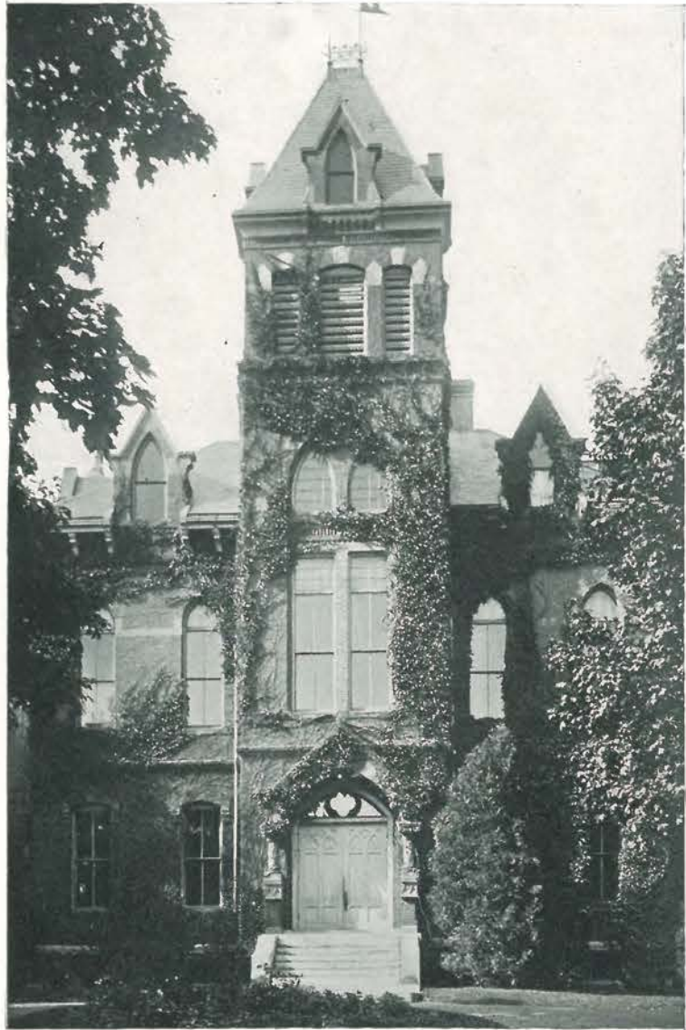
ENTRANCE TO CORTHELL HALL
