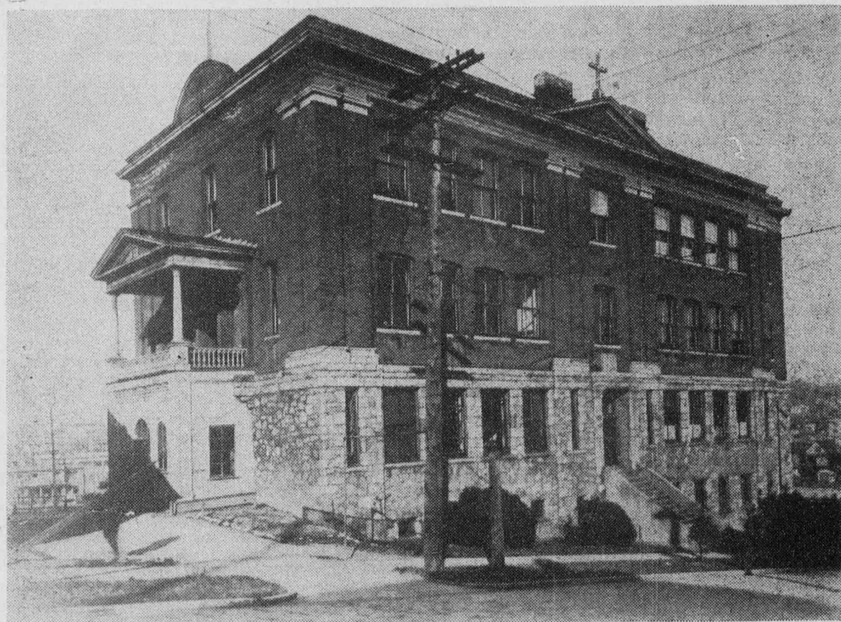
This is the Marion Street side of the Science Building as it appeared after repairs following the 1907 fire. Note the roof has been flattened and the steeple removed.
