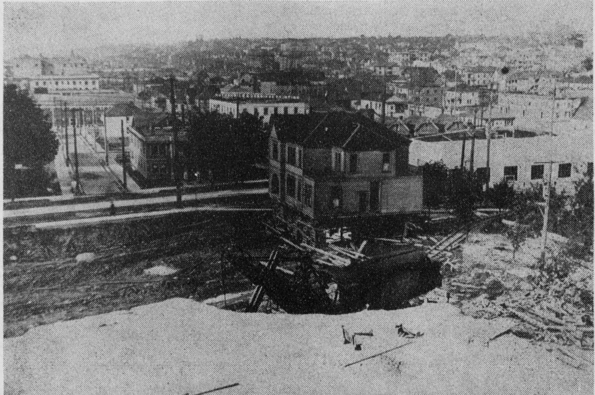
The old WCTU building ready to be lowered to its new site. Note the old car barn, now Seattle University's Engineering Building, which currently is having "a facial."
