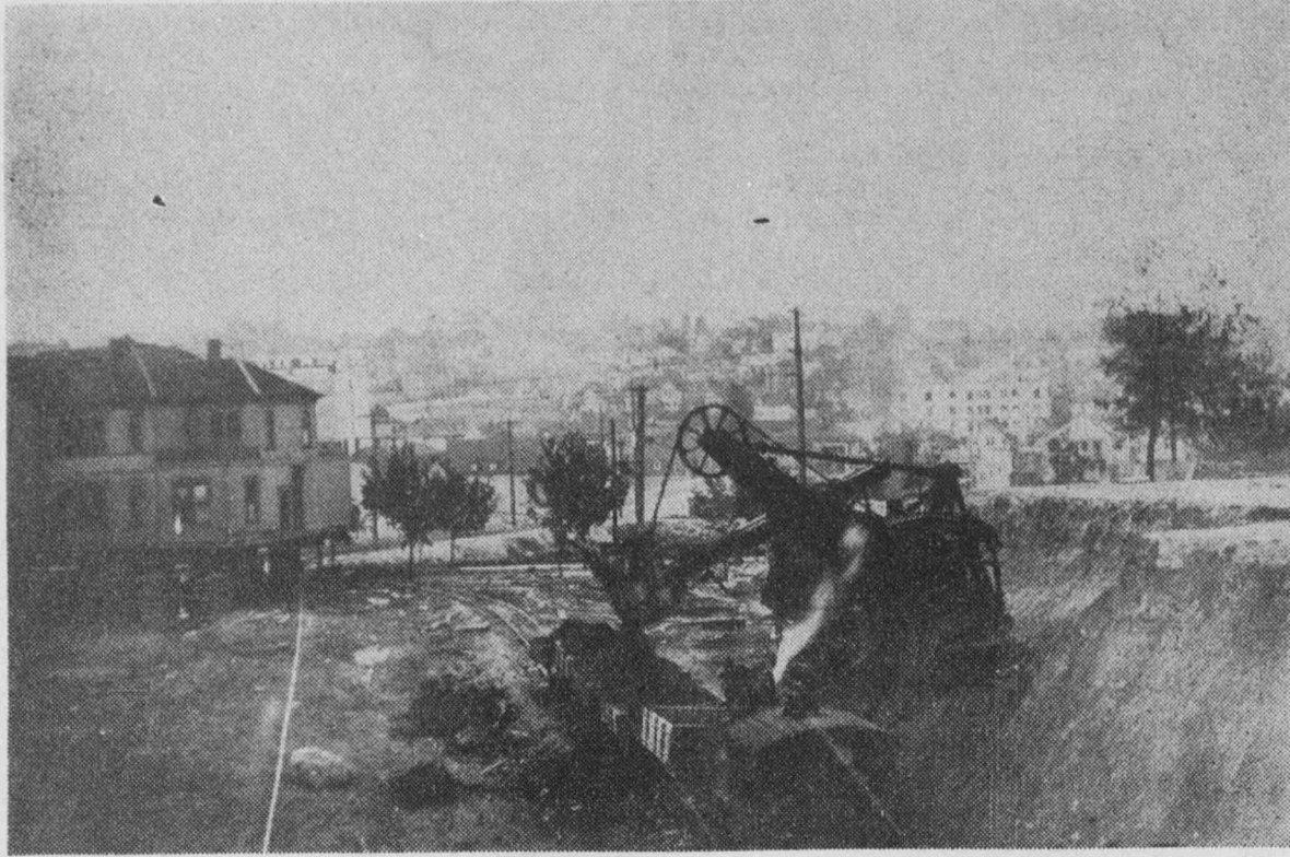
This picture of excavators at work was taken from Marion and Broadway. The old WCTU nursery was being moved to Eleventh and Madison, the spot now occupied by the south wing of the Liberal Arts Building.
