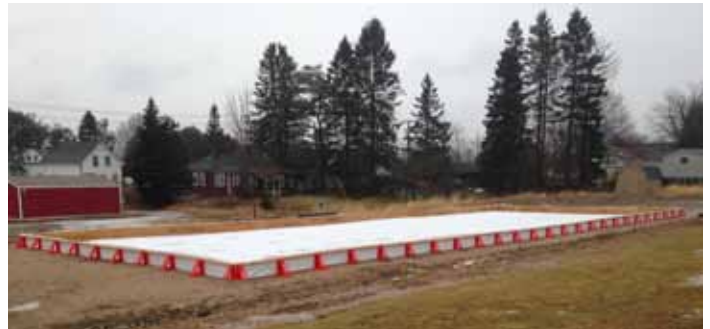
DCF public restitution crews installed an ice skating rink in the Town of Machias.
