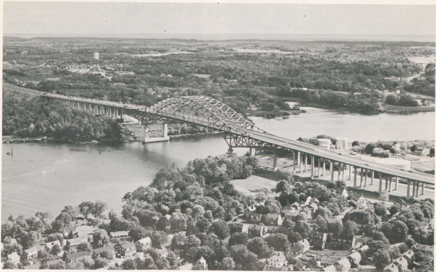
Piscataqua River Bridge as seen from over Portsmouth, New Hampshire, looking towards Kittery, Maine.
