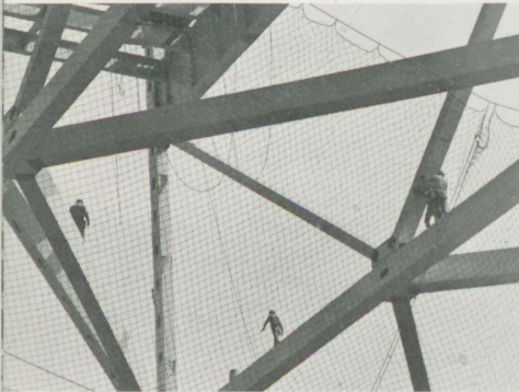
Ironworkers assembled 10,000 tons of steel high over the river.
