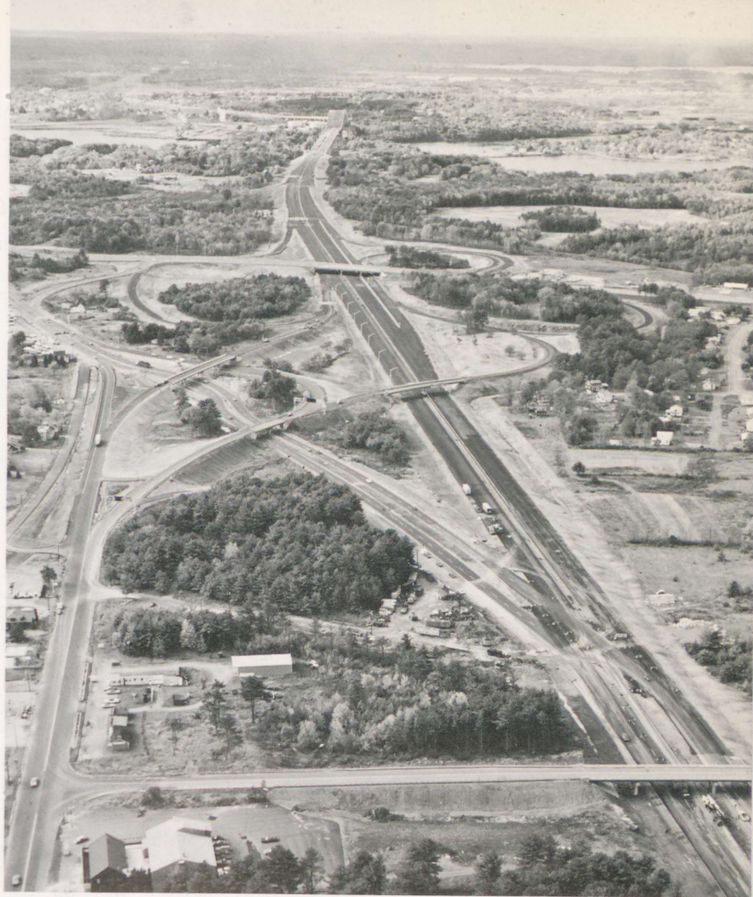
Maine's I-95 approach looking towards the south with Route 101 in the foreground, Route 236 interchange in the center, the bridge is beyond.
