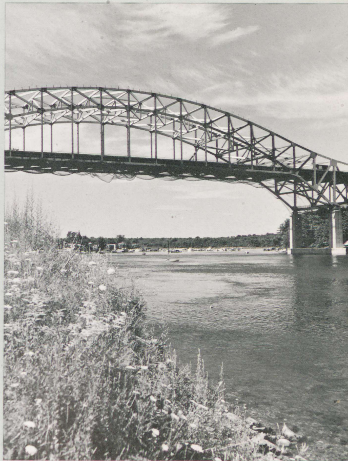
The big bridge during final stages of construction.
