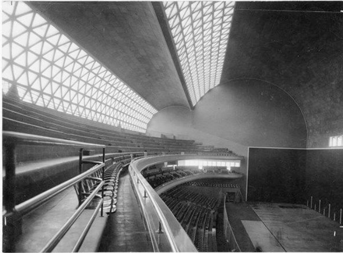
Fig. 4: Interior view of the roof of the Recoletos Fronton. Eduardo Torroja 1935. Madrid. Spain.
