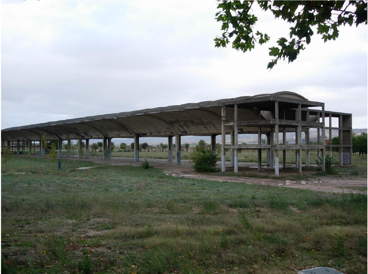
Fig. 6: Current status of hangars.
