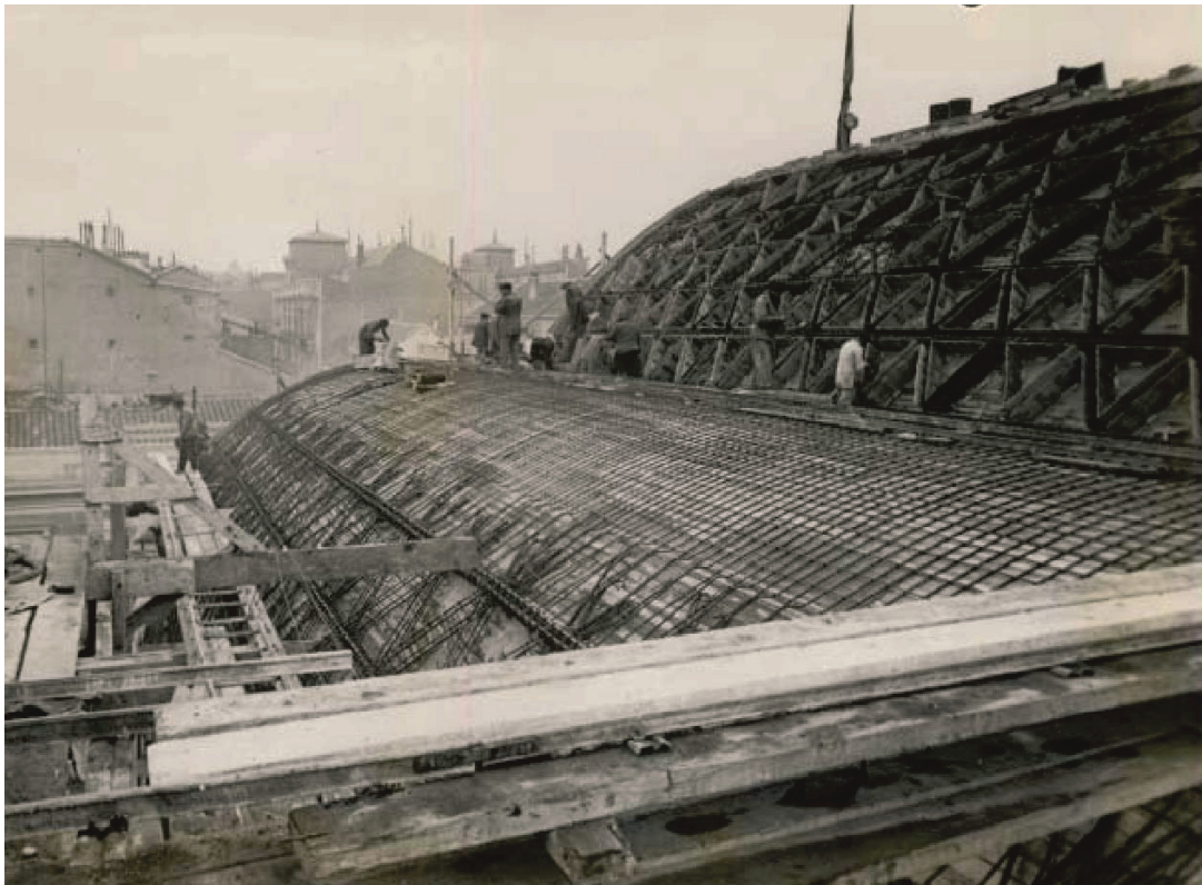
Figure 2. Preparing the steel
