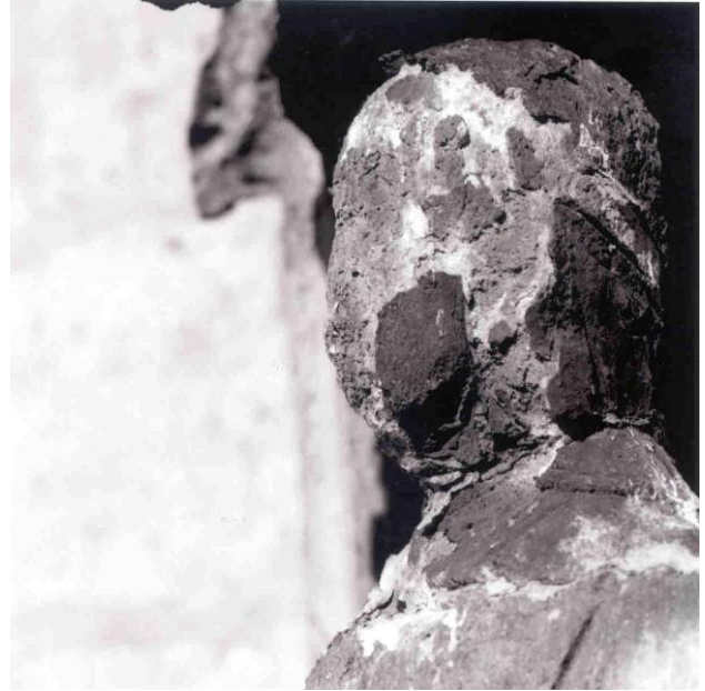
Fig. 3. State of conservation of some sculptures completely ruined due to the water and external agents
