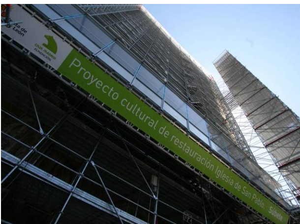
Fig. 12. The lift platform for the public that permitted to visit the restoration works on the façade
