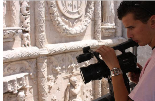
Fig. 13. Recording the façade with video from the lift platform once the restoration works have finished
