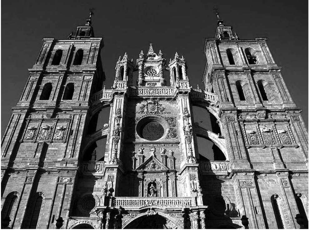
Fig. 16-Astorga, cathedral façade, XVIII century restorations; towers' remates from XIX and XX century.
