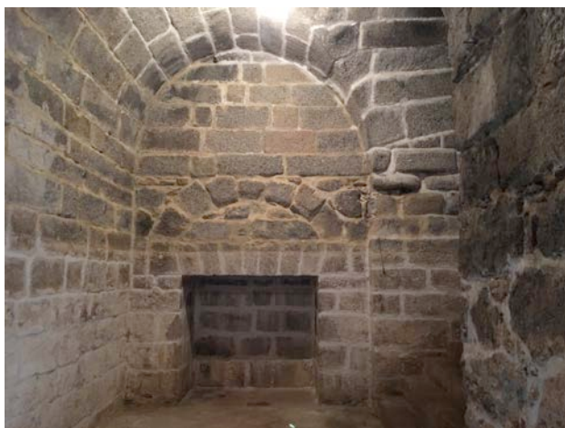
Figure 12. The geometry and stereotomy of the inner vaults and their intersections evidence a construction with a varied repertoire of solutions and techniques.
